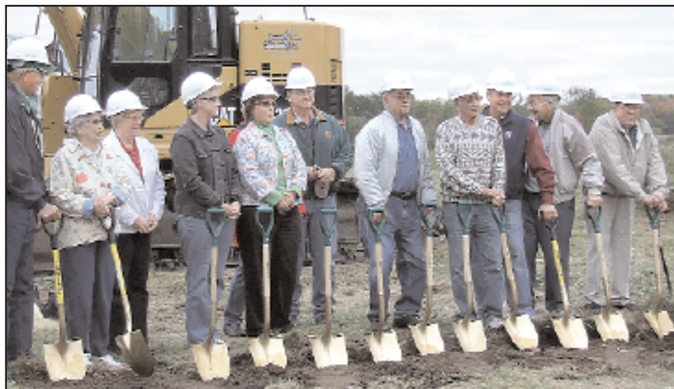
Turning over the first spades of dirt for the new UPH building project were current and past board members. Shown (L to R) are board member Wayne Shirley, former UPH administrator Edna Lawson, former board members Marlys Pederson and Mary Jo Nelson, board members Nora Asper and Craig Adair, with Marie Bazey behind, board member Irvin Hermstad, board President Dick Coen, board member Mike Broten, and former board members Gayland Jensen and Edwin Pedersen.
