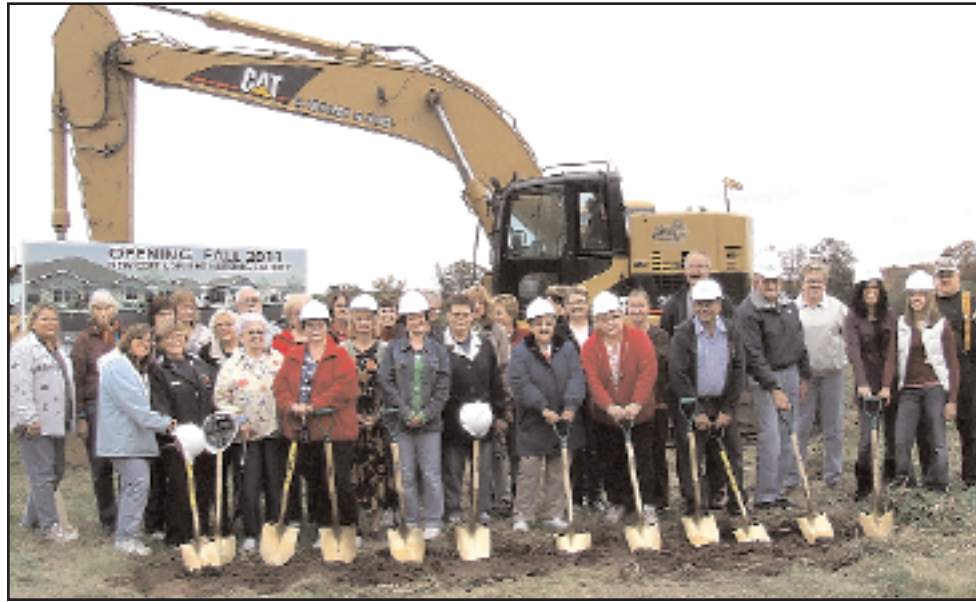
Former and current staff pose with hardhats, shovels, and excavating equipment to celebrate the groundbreaking for United Pioneer Home's new building. — Photos by Mary Stirrat
